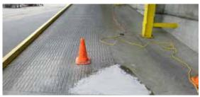
The Belzona 4151 + 4111 system was used to rebuild and smooth the cracked area
