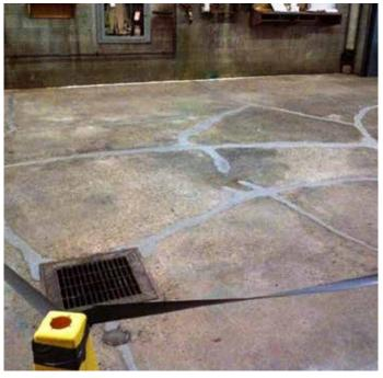
Crack repaired with Belzona 4151 and 4111 system
